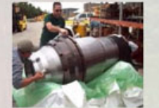
Liquid Rust Removal
