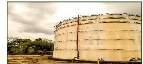
VCI, can be used for the protection of aboveground storage tank bottoms from soil-side corrosion.
